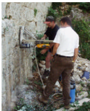
Drilling and taking samples at abutment west
